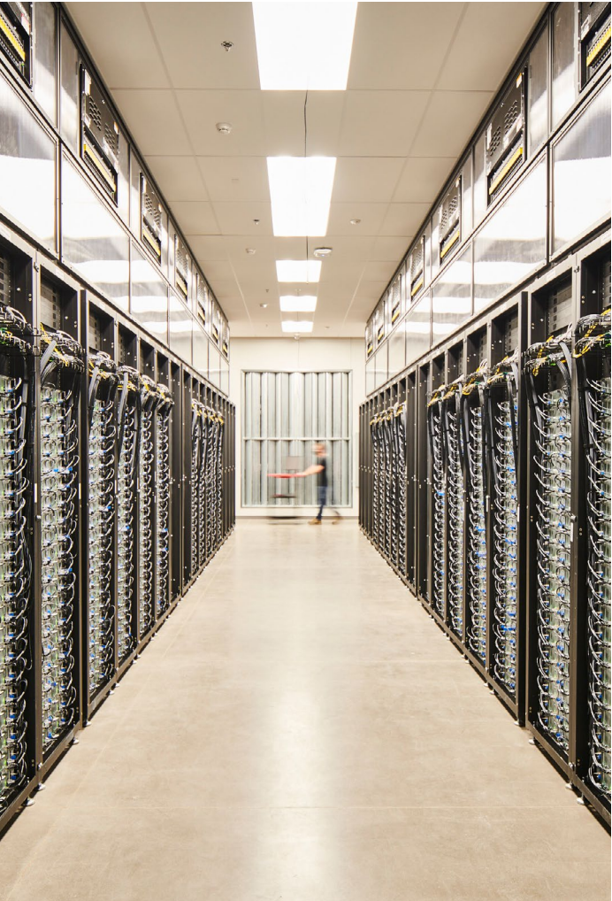
Apple’s Reno data center, opened in 2012, takes advantage of the mild climate by cooling its servers with outside air whenever possible.
